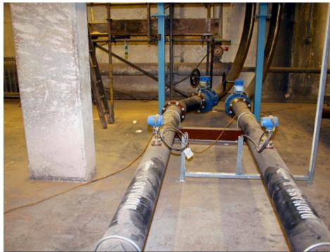
Need to bypass coal mills Present the fuel to the boiler as powder In house – 20T/hr direct injection system
