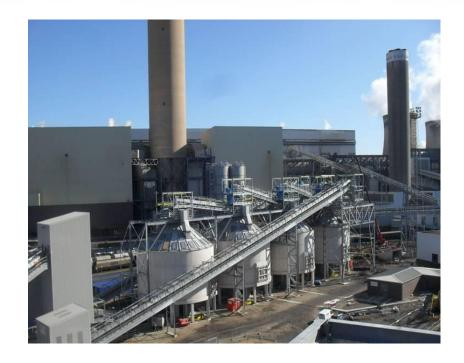
20 t/hr pilot facility success leads to 1.5t pa facility with road and rail receipt and 24,500t storage R&D issues around safety, storage handling, transport, sampling
